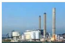
Thermal Power Plants
